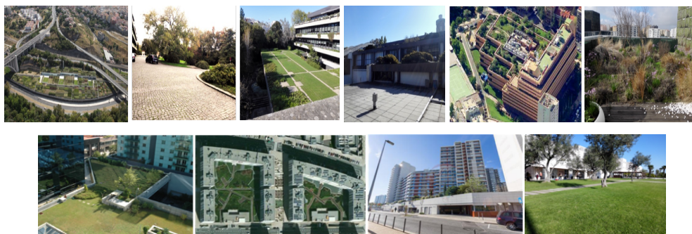
Figure 2. Green roofs of the inspected case studies I, II, III, IV, V, VI, VII, VIII, IX and X (from left to right).
